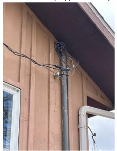
The overhead service wires are deflected by trees. We recommend the trees be trimmed clear of the wires or the service be reconfigured. To reduce shock hazard during this procedure, the work should be coordinated with the utility provider.
