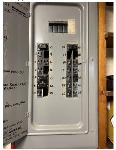
The circuits in the panel are labeled. We did not verify the accuracy of the labeling, but it appears to be typical. When the opportunity arises, we suggest checking the labeling by actually operating the breakers.
