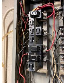
There are holes in the service panel where 'knockouts' have been removed and left open. This is not an approved practice and we recommend the holes be closed with approved filler plates.
