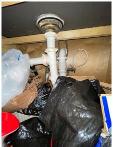
The drain trap has been installed in a substandard manner. We recommend it be repaired or replaced.
